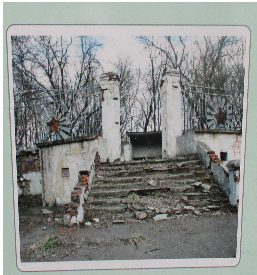
State of disrepair of park pavilion
